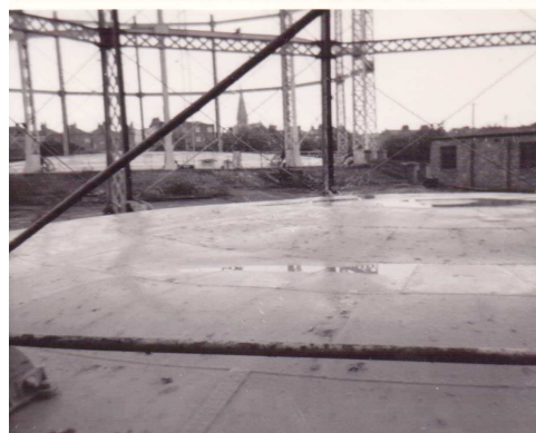
Kings Road Holders awaiting demolition
