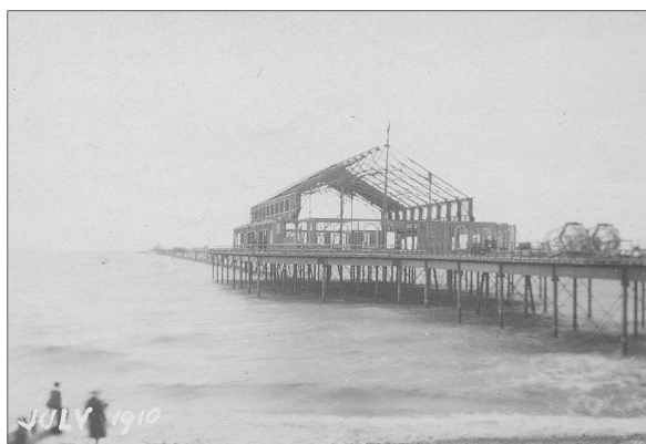
Building work in progress
