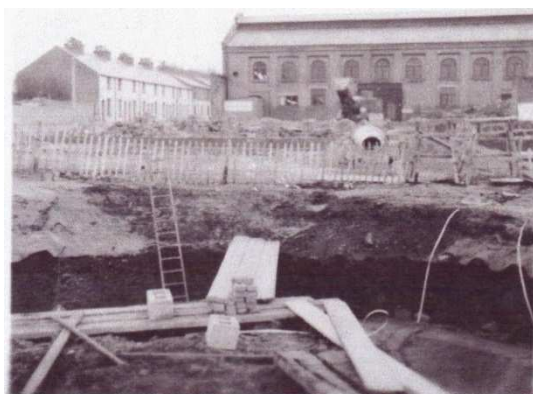
Holder site being excavated for Jacksons Garage
